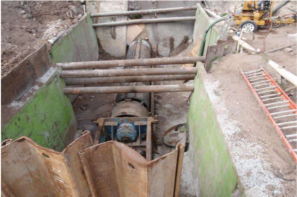
UNDERGROUND INSTALLATION JACK AND BORE EXAMPLE
